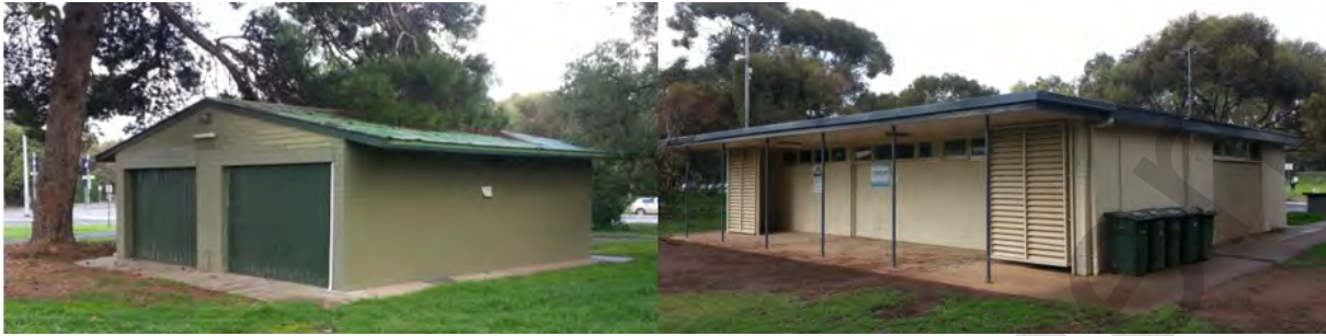
Existing Buildings in Park 9
